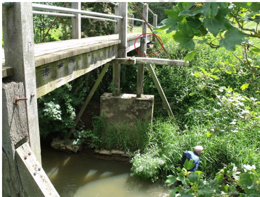
Underwater inspection in progress, SR497 Penshurst
